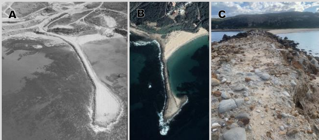
Figure 4. Photos of Mawsons Breakwater after construction in 1970 (A), in 2019 (B) and 2020 (C) Sources: (A) Hilder Collection, Hunter Photobank Newcastle Library; (B) Google Earth; (C) P Dwyer
