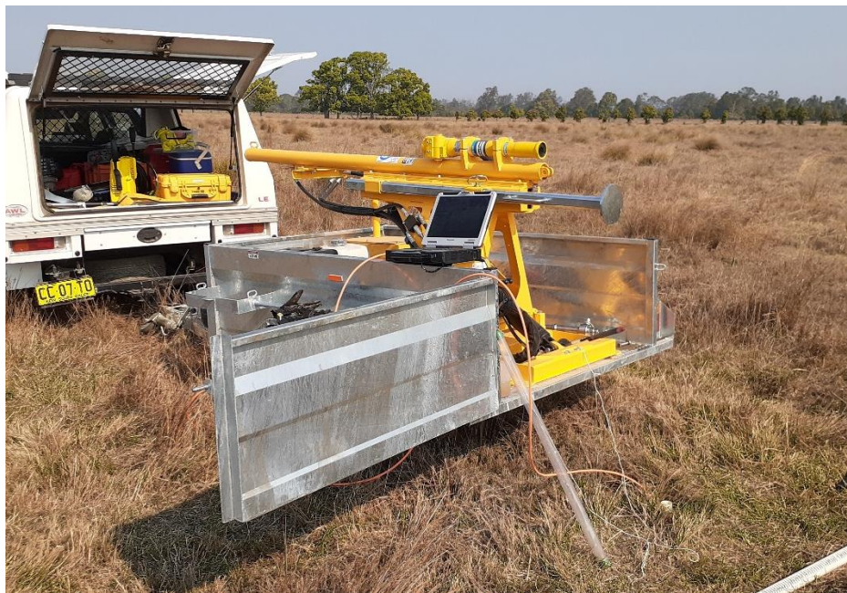
Figure A.11: A field computer connected to a water level logger (via the orange cable) to measure the recharge rate following a removal of a slug of water from the temporary borehole
