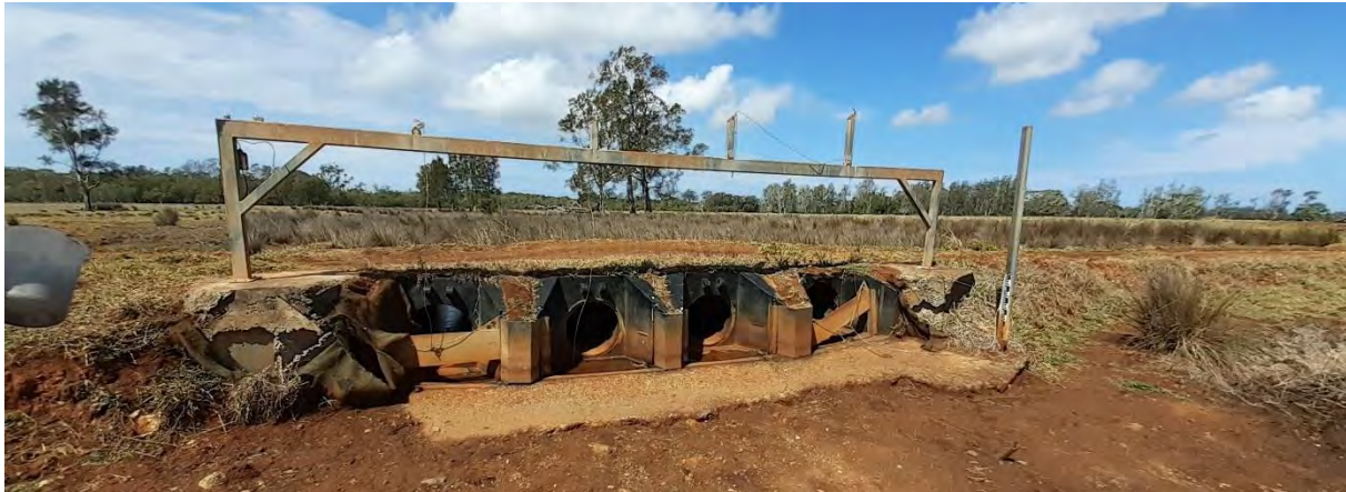
Figure 8-54: ID ASSS_17 - pipe culvert with dropboards (not in place)
