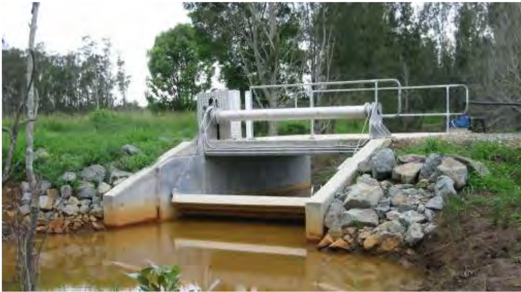
Figure 8-23: ID ASSS_01 hinged weir (Source: Hastings Council (2004))
