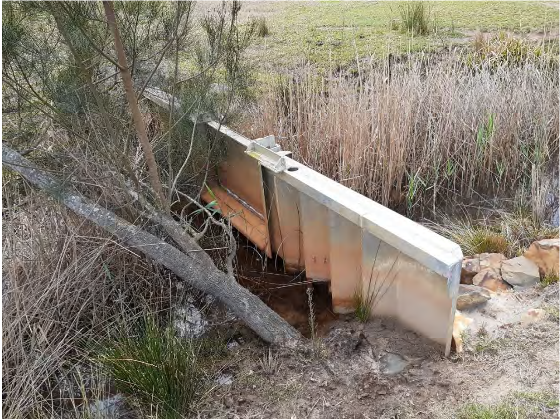
Figure 8-5: Example of a floodgated weir at ASSS_40 on Torrens Island
