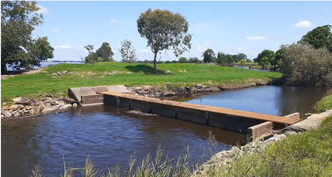
Figure 8-83: Alummy Creek Weir on Southgate Creek (sluice gates in place)
