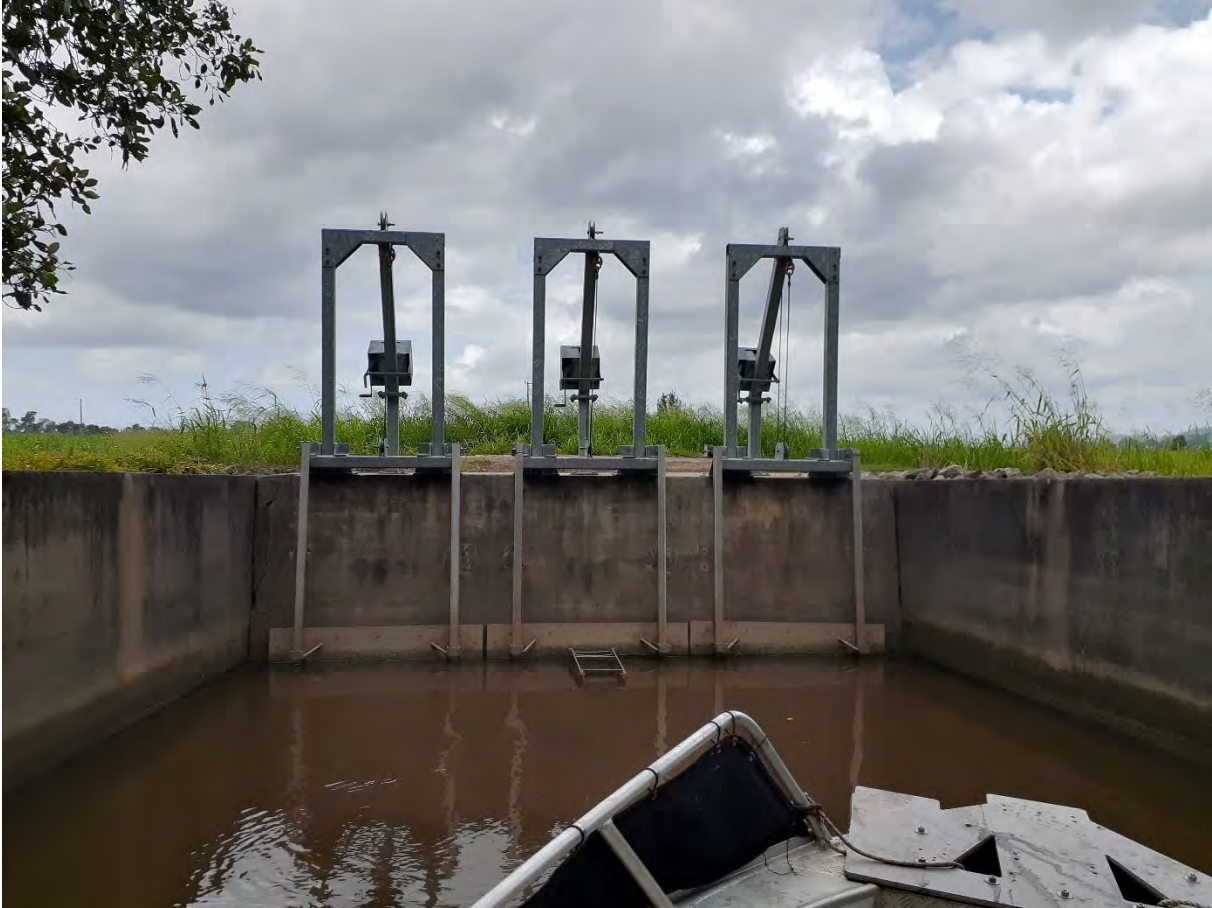
Figure 8-47: F-2560-FB-0001 with a buoyancy gate on the middle floodgate, and lifting device on all three floodgates
