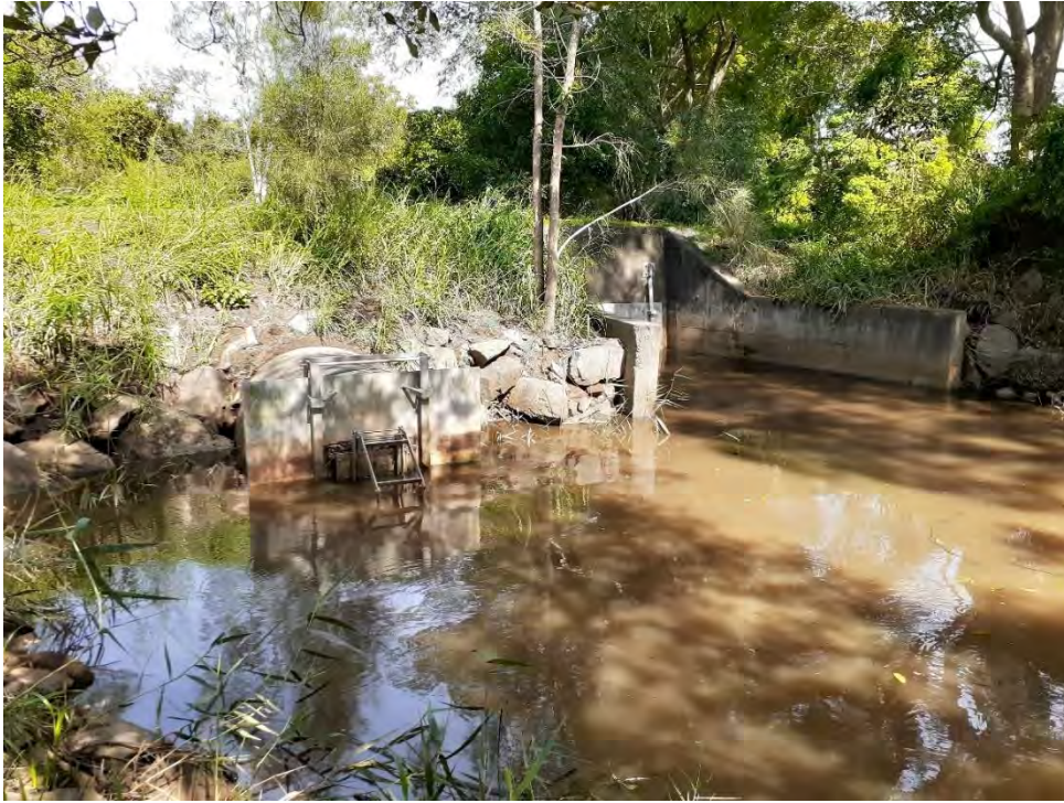
Figure 8-79: Secondary floodgate with buoyancy gate at floodgate ID F-2400-FT on Poverty Creek
