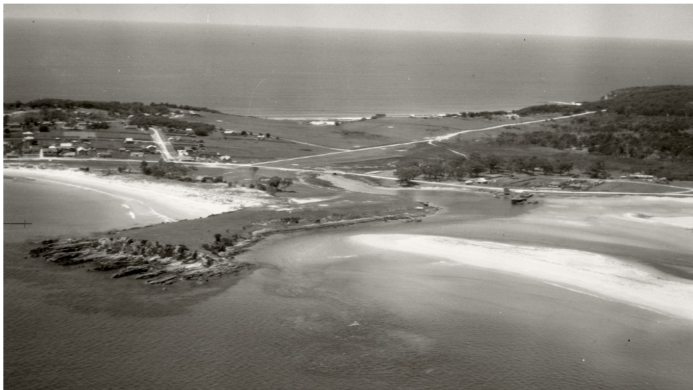
Aerial photo from November 1937 showing the natural condition of the entrance to the Bermagui River prior to the installation of breakwaters, training wall and estuary harbour infrastructure
