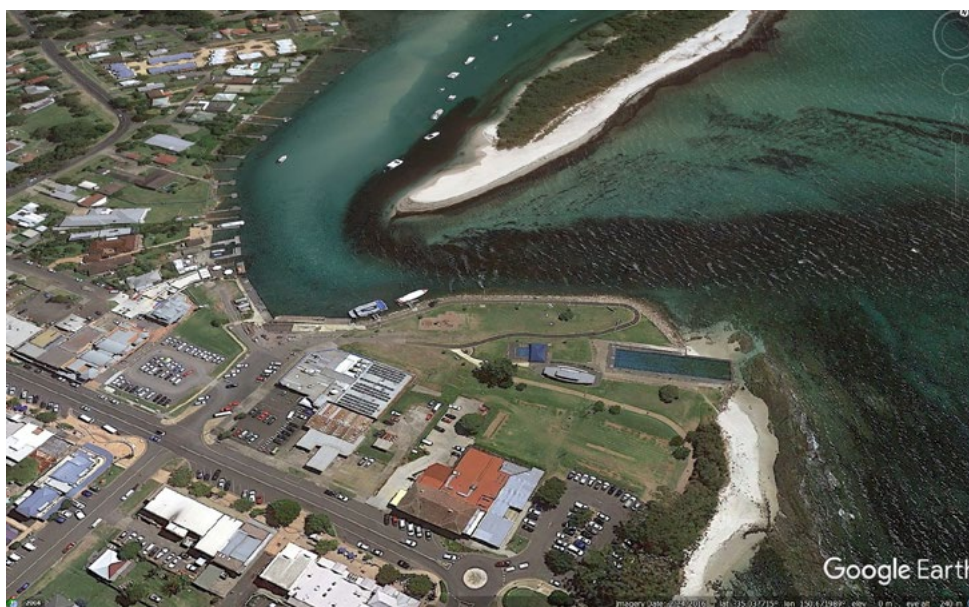
The Currambene Creek breakwater and the Huskisson Ocean Pool built in 1965. Credit: Google Earth
