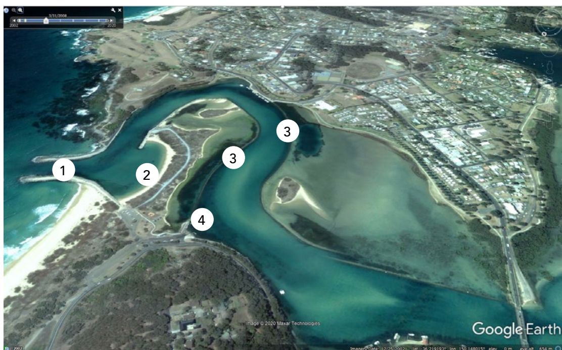
The Wagonga River estuary and its breakwater and trained entrance showing: (1) entrance breakwaters; (2) wave-trap beach; (3) estuary training walls; (4) heritage lock built in 1939 to pen Eastern Australian Salmon. Credit: Google Earth
