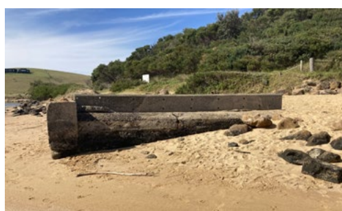
Part of the deteriorated and buried concrete race and pipeline at the entrance to Werri Lagoon in 1970s (LHS) and today. Credit: Kiama Council and Byron Robinson
