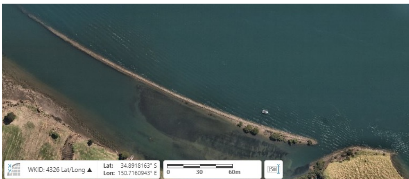
The training wall at Numbaa Point installed to address some of the erosion occurring in Berrys Canal in the early 1900s Credit: nearmap
