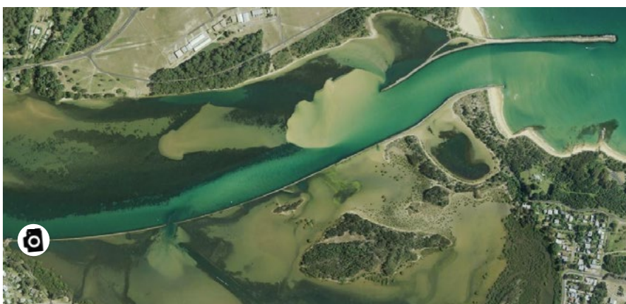
The Moruya River southern breakwater and training wall
