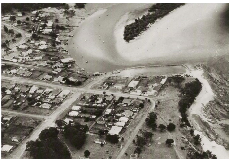
In 1961, the trained entrance of Currambene Creek incorporated an estuarine swimming enclosure that was later infilled to create parkland. Source: Crown Lands
