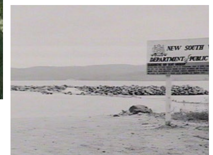
Quarantine Bay, Eden: breakwater and launching ramp, 1979
