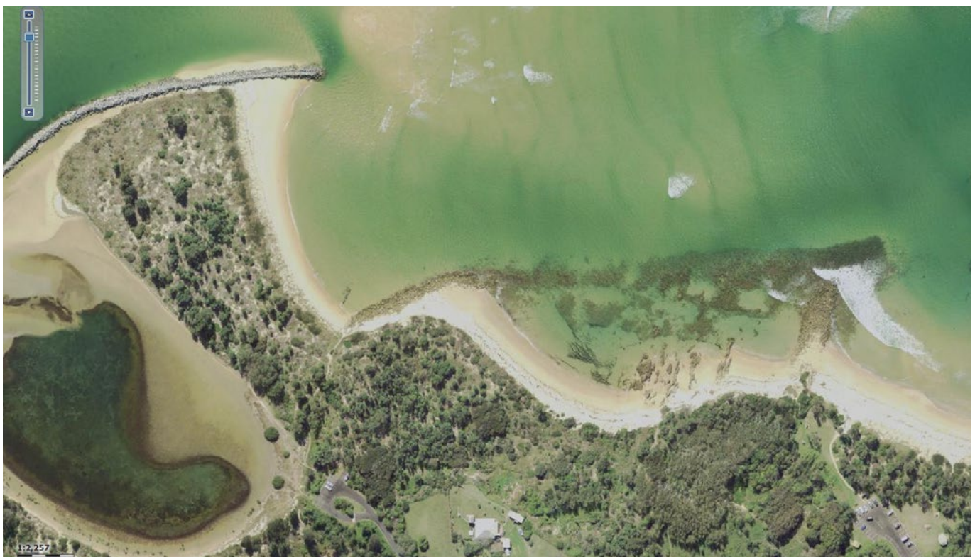
The Moruya River southern breakwater and submerged remnants of the original, heritage listed, southern breakwater. Credit: Six Maps
