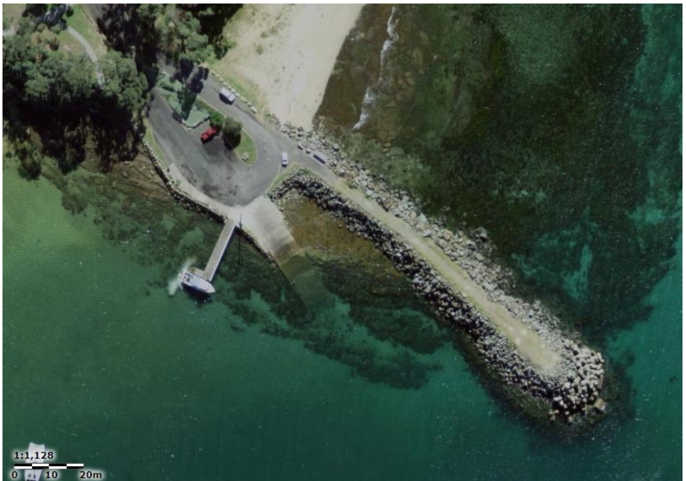
The Ulladulla Harbour northern breakwater Credit: Six Maps
