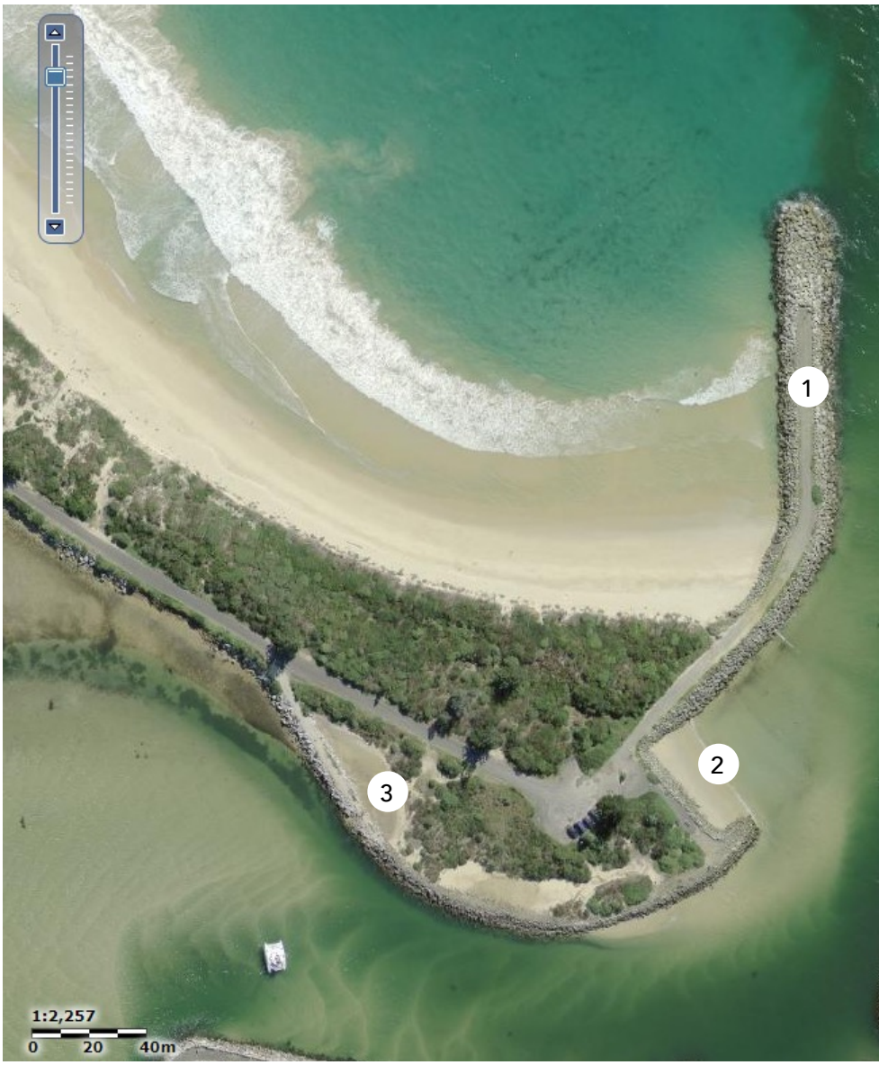
The Bermagui River northern breakwater: (1) northern breakwater; (2) northern wave-trap beach; (3) an area where tidal flows through the training wall create an intertidal that could be enhanced for a small area of fish or bird forage habitat Credit: Six Maps
