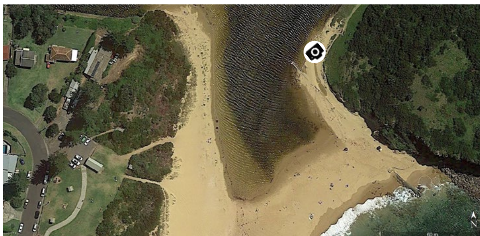
Entrance of Werri Lagoon, Gerringong with the concrete training pipe on the northern bank Credit: Google Earth
