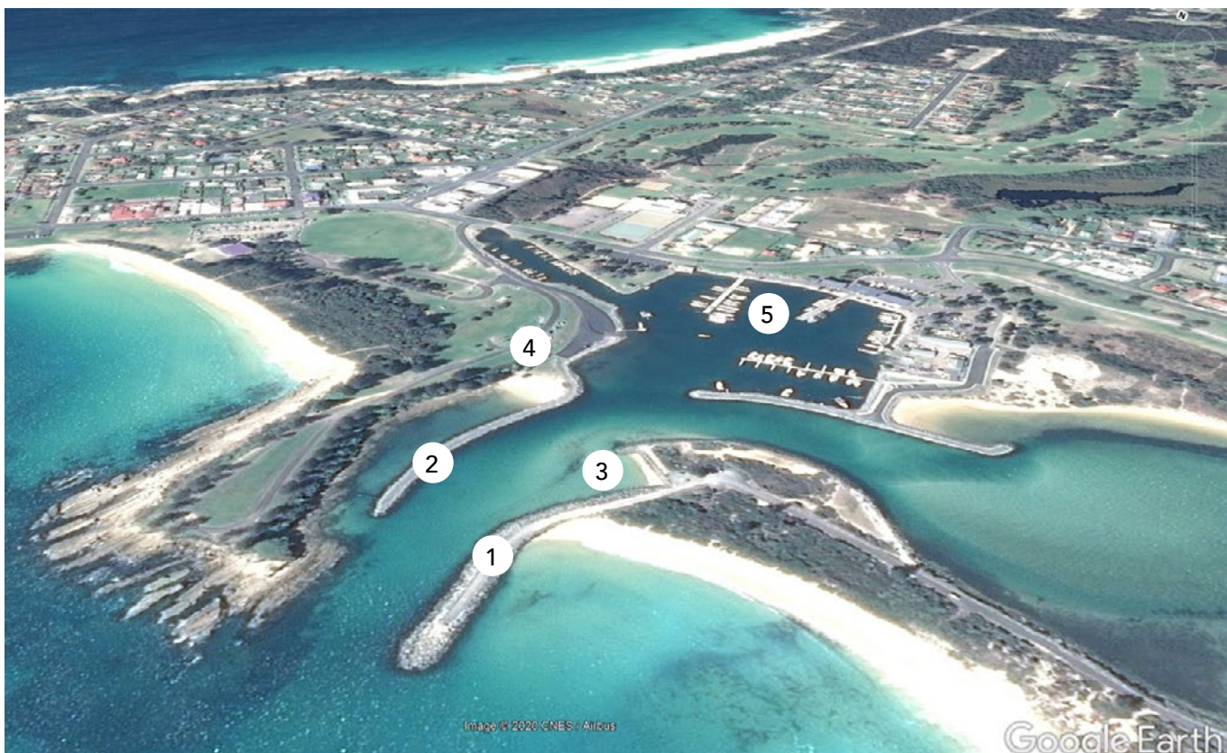
The Bermagui River estuary and its trained entrance: (1) northern breakwater; (2) southern breakwater; (3) northern wave-trap beach; (4) southern wave-trap beach; (5) Bermagui Harbour Credit: Google Earth
