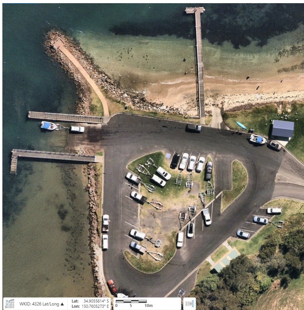
The Crookhaven regional boat ramp and breakwater
