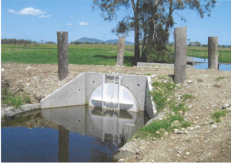
Figure 8-45: Floodgate on Kinchela No. 2 Drain (Source: Ron Kemsley, Kempsey Shire Council)
