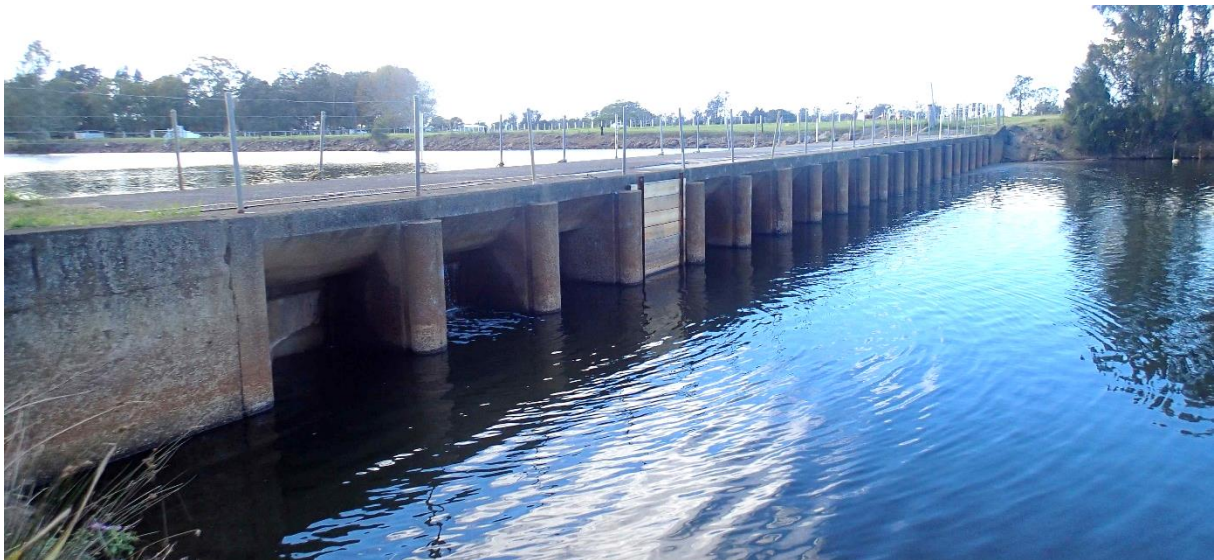
Figure 8-2: Menarcobrinni floodgates (Rayner et al., 2020)
