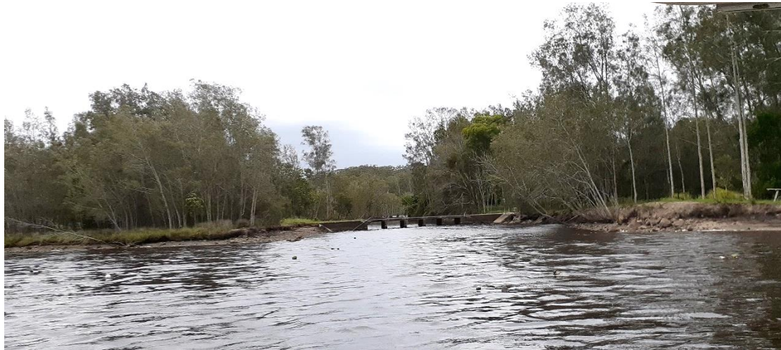
Figure 8-23: Structure 009G1 allowing full tidal flow between Yarrahapinni Broadwater and Andersons Inlet (March 2020)
