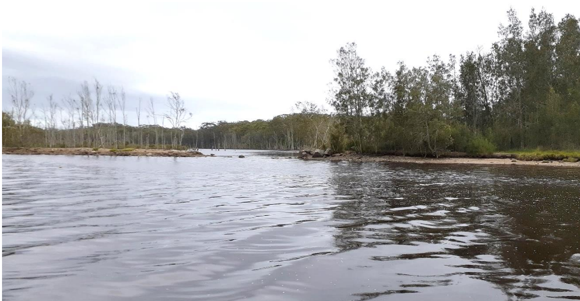
Figure 8-24: A breakthrough in the levee allowing tidal exchange between Yarrahapinni Broadwater and Andersons Inlet (March 2020)
