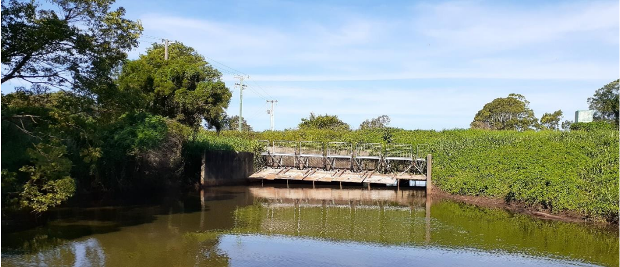
Figure 8-32: Belmore River headworks (017G1) winched open when inspected in March 2020
