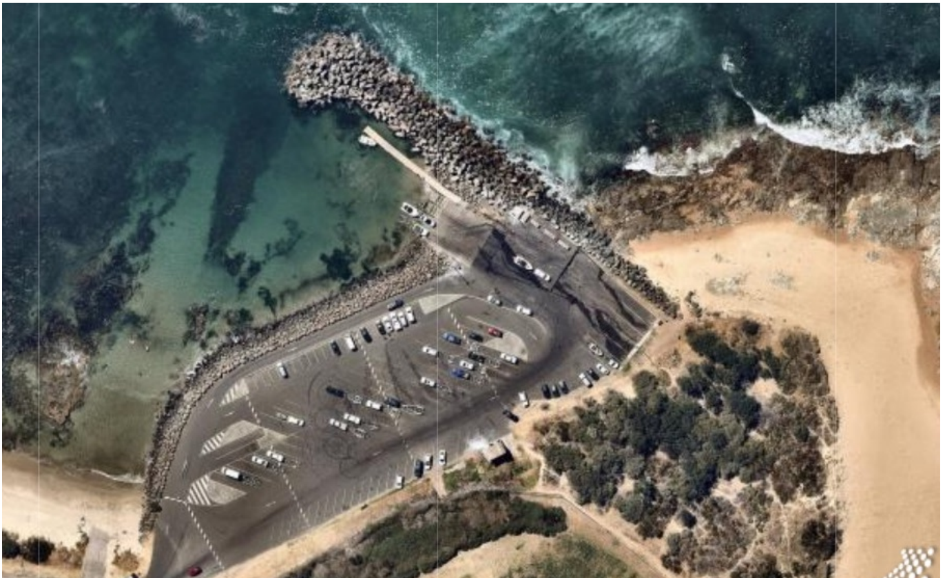
The Bellambi Point breakwater, boat launching ramp and carpark Credit: nearmap
