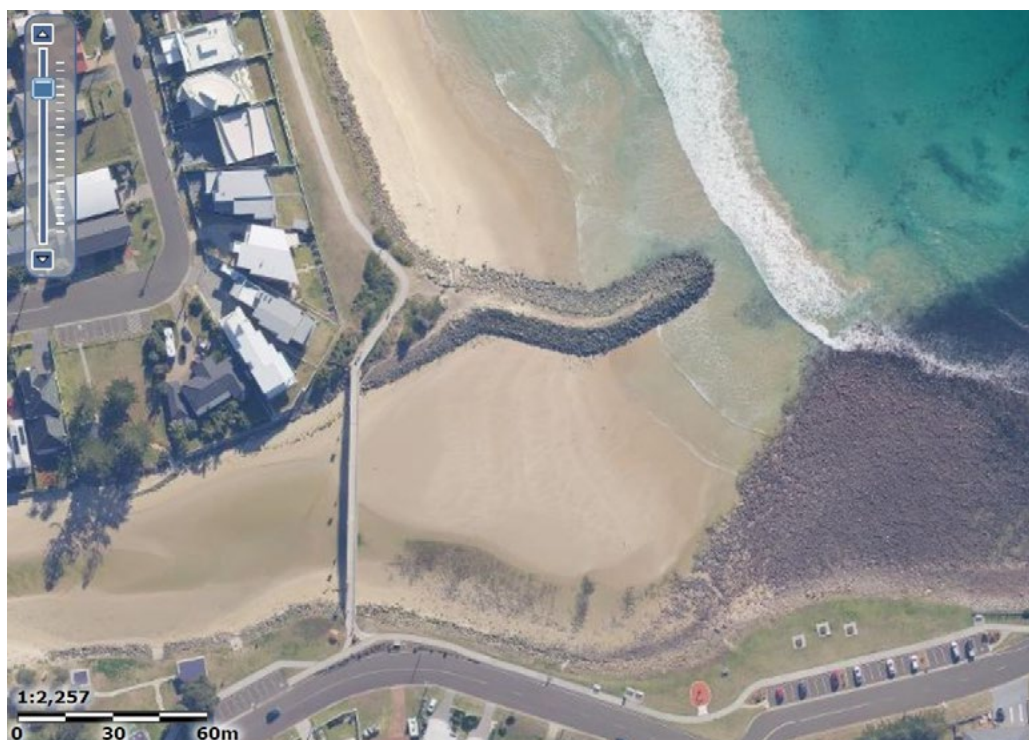
The Barrack Point training wall was extended in 2006-08 Credit: Six map
