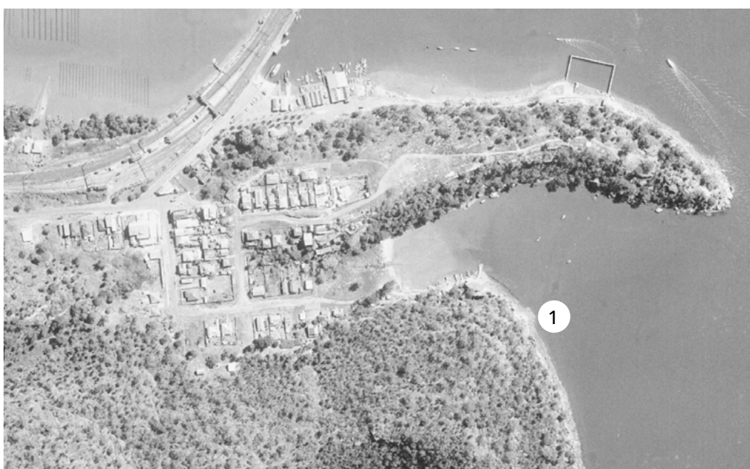
Parsley Bay Breakwater at Brooklyn, Hawkesbury River showing (1) the location of the breakwater in 2018 (above) and in 1961, prior to the breakwater being installed circa 1965 (below). Part of the bay has also been reclaimed for the carpark and foreshore facilities Credit: Crown Lands and Google Earth
