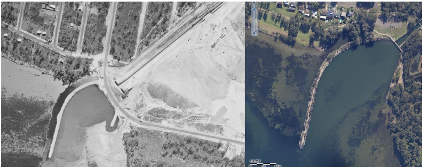
The San Remo breakwater at Budgewoi Lake directs water releases from the Colongra gas-fired power station into Budgewoi Lake. The images show the breakwater in 1965 (left) and 2017 (right) Credit: Crown Lands and Google Earth
