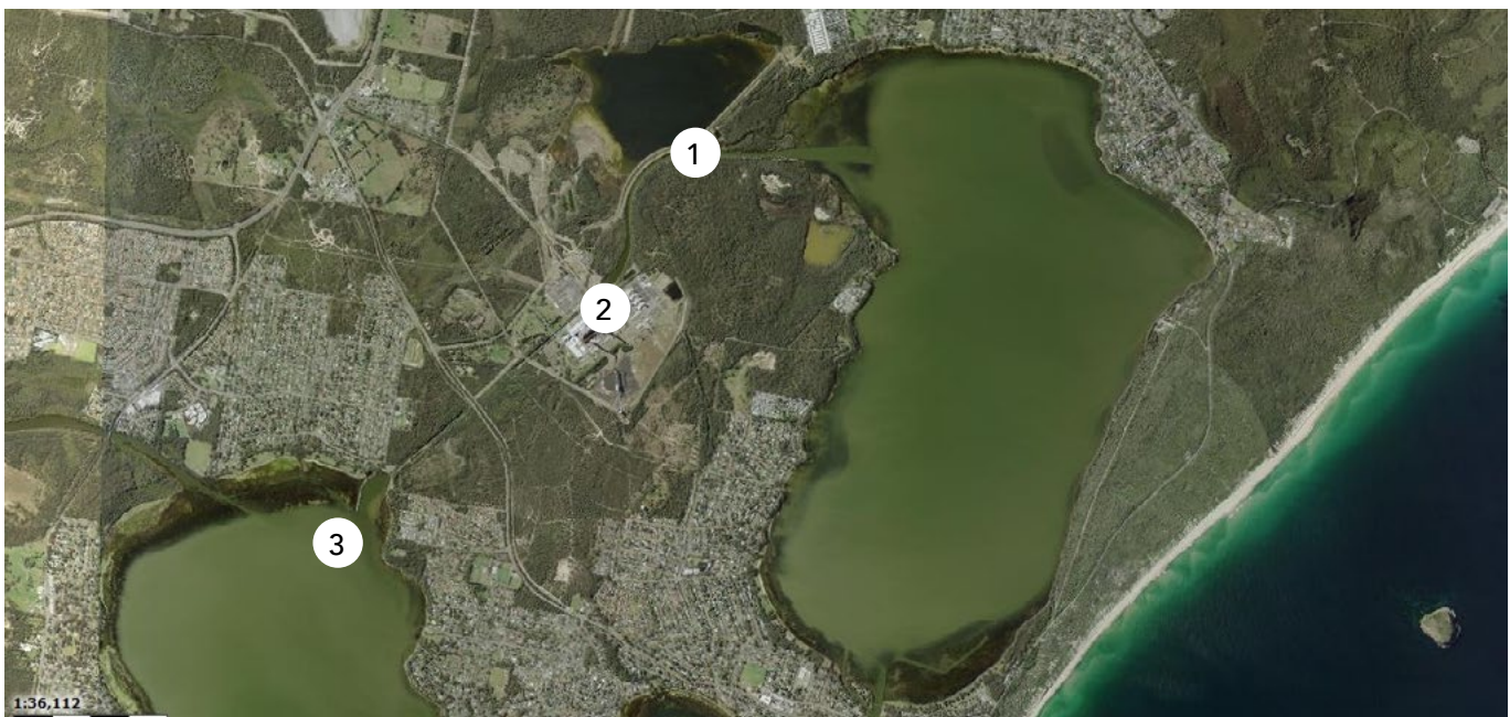
Water from Lake Munmorah is drawn into an intake (1), used at the power station (2) and released into Budgewoi Lake (3)
