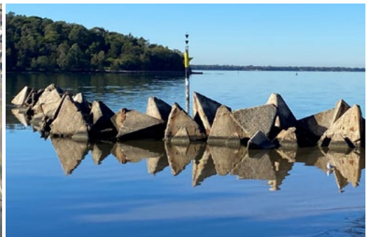
Repurposed tank trap tetra-hedrons used to form the original breakwater are still evident in the structure Credit: Carla Ganassin
