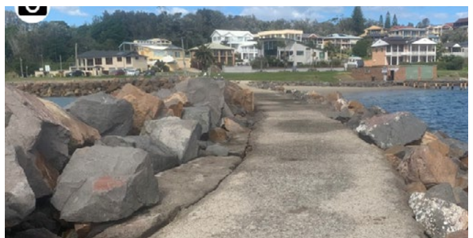
The rubble crest surface of the southern breakwater and the concrete surface of Lucys Groyne
