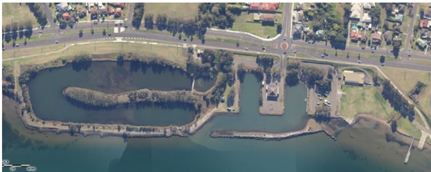
An area adjacent to Berkeley Harbour was reclaimed and then manipulated to improve water quality from Budjung Creek Credit: Six Maps
