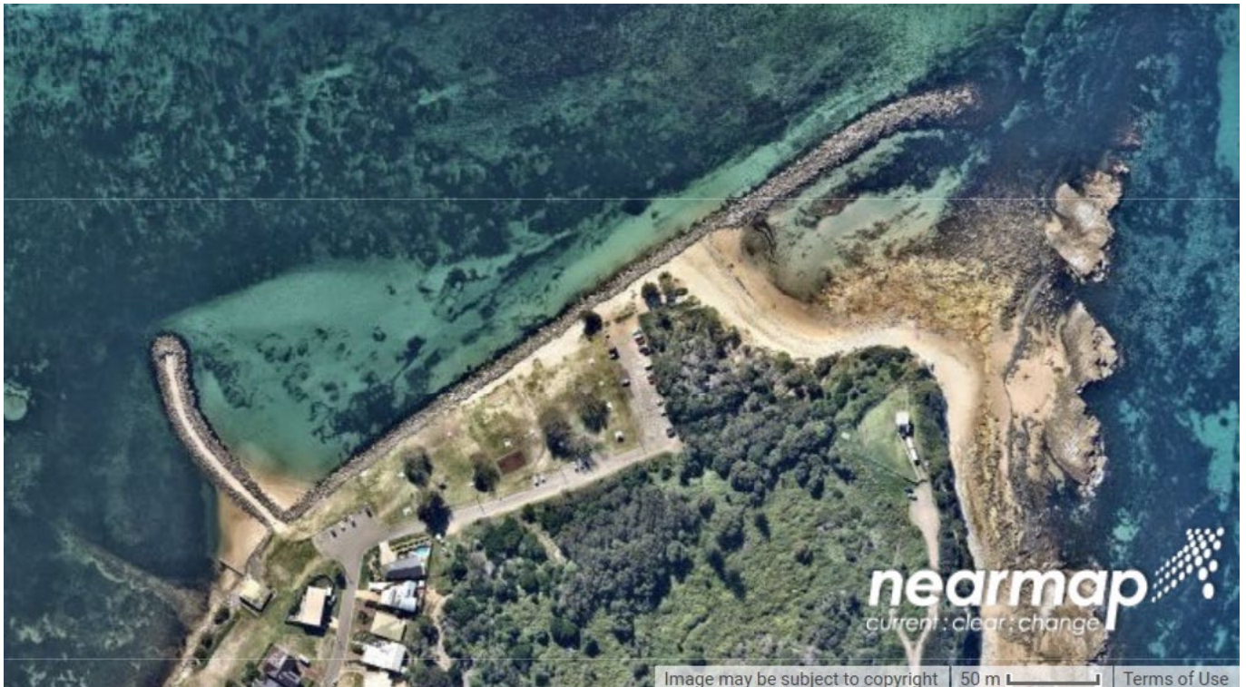
Aerial photo of (1) the Lake Macquarie southern breakwater (2) Lucys Groyne and (3) remnant erosion protection works Credit: nearmap
