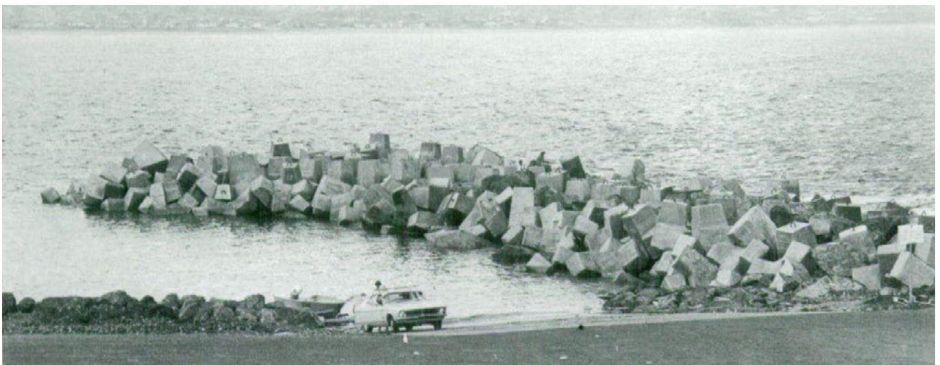
Bellambi Point ocean breakwater protecting a boat ramp Source: NSW Public Works Department Annual Report 1980
