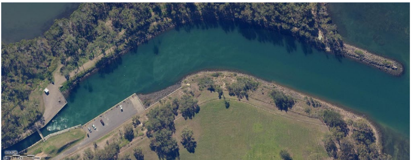
The breakwater at the Eraring Power Station cooling water outlet Credit: Six Maps
