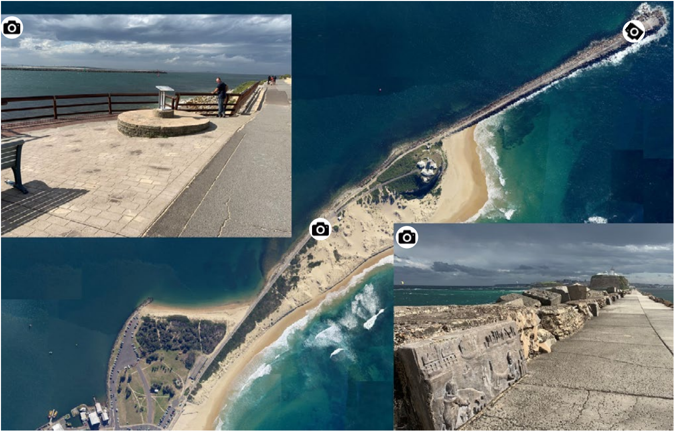
The Hunter estuary southern breakwater showing seating opportunities and relief artwork used to explain the historical importance of the breakwater Credit: Google Earth
