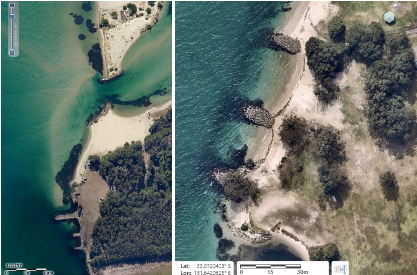
Detail of Swan Bay entrance in 2013 after groynes were used to narrow the entrance to the Bay (left) and control erosion downstream near Pelican Inlet (right) Credit: Six Maps
