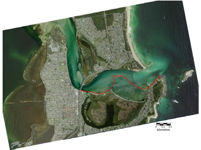
The foreshore around the entrance has retreated since 1914. The parish map (left) and the red line of the 2018 aerial photograph (right) show the original shoreline. Credit: Six Maps
