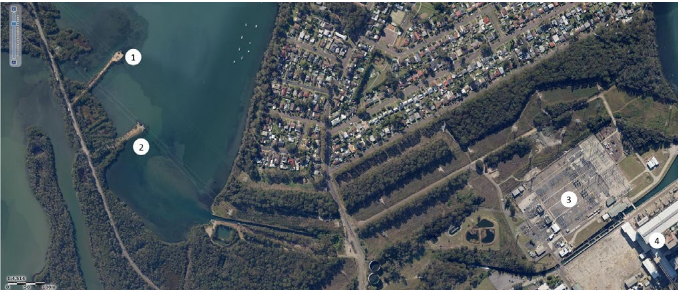
Manning Point breakwaters, installed as part of the powerline infrastructure for the Vales Point power station in 1965 (above) and 2017 showing (1) the original breakwater; (2) second breakwater also built in the 1960s; (3) electricity substation and (4) Vales Point Power Plant Credit: Crown Lands and Google Earth
