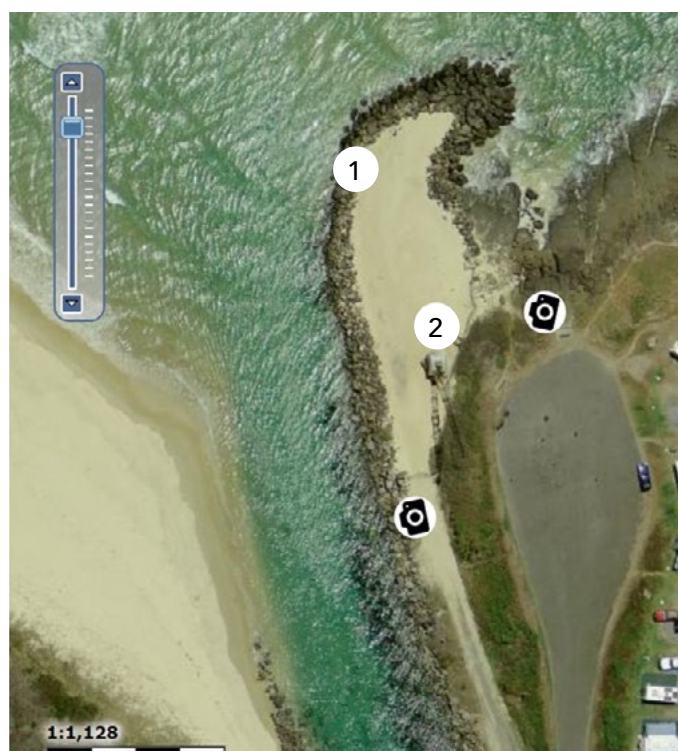
South West Rocks Creek southern breakwater: (1) the southern breakwater; (2) dredge drag-line crane Credit: Six Maps
