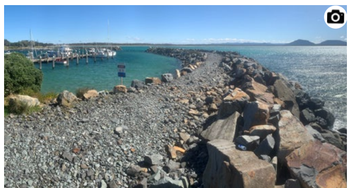
Rubble crest surface on the Crowdy Bay eastern breakwater
