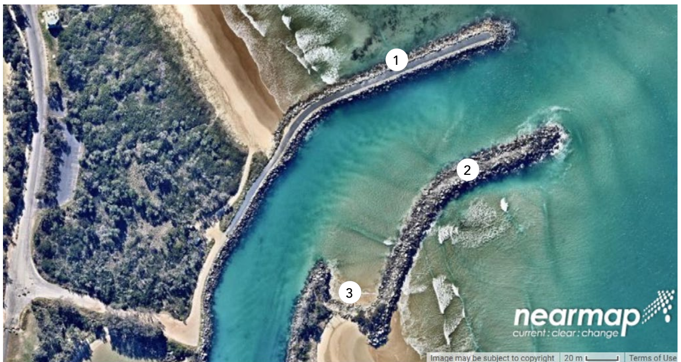
Aerial photo of the Wooli estuary showing (1) northern breakwater; (2) southern breakwater; (3) wave-trap beach
