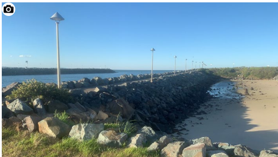
The backwater wading pool relies on tidal flows filtering through the breakwater
