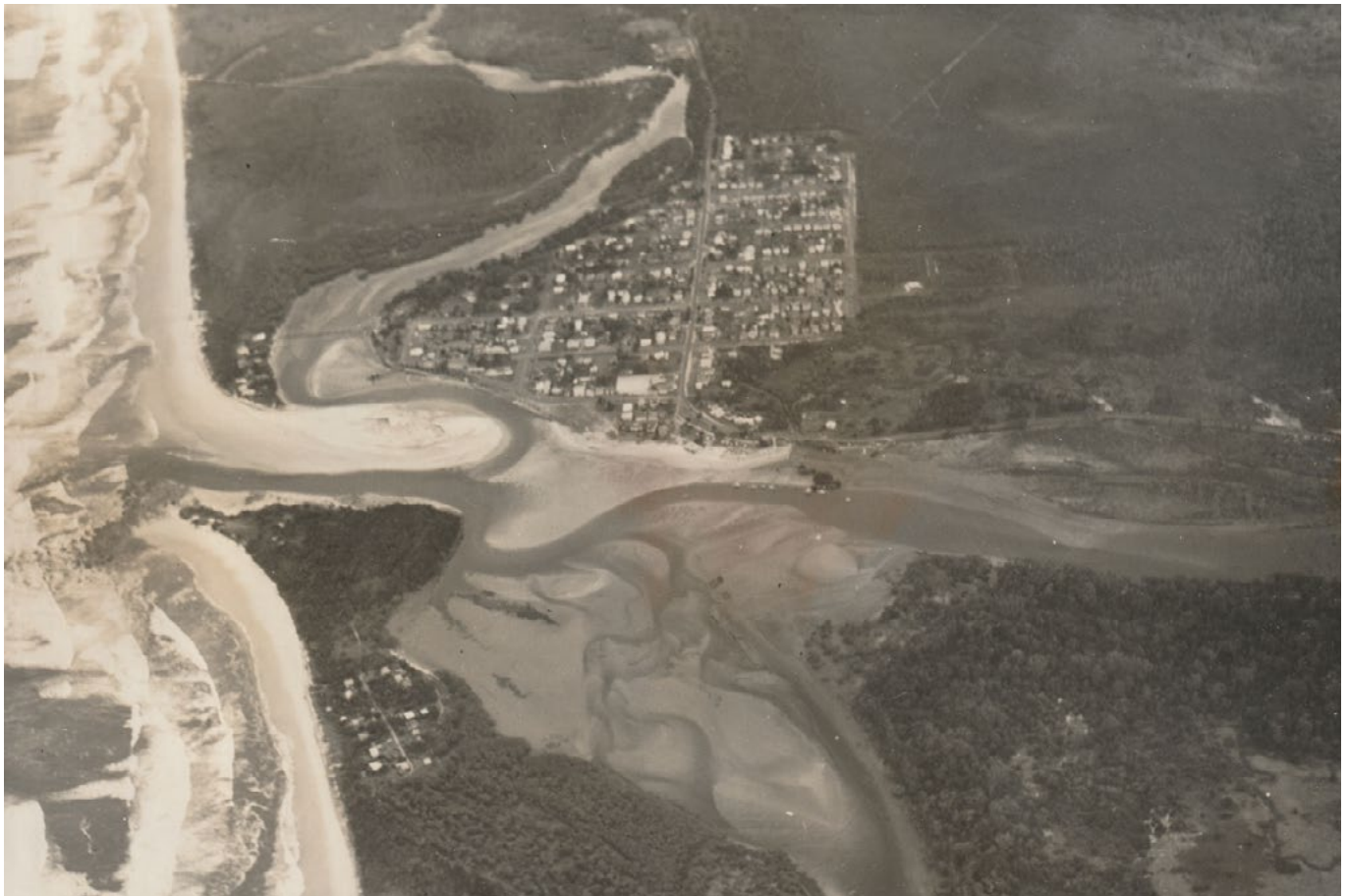
Aerial photo of the Brunswick River estuary looking south, April 1960, before the breakwaters were installed. The village of Sheltering Palms on the northern side of the Brunswick River was abandoned in 1975 due to coastal erosion.
