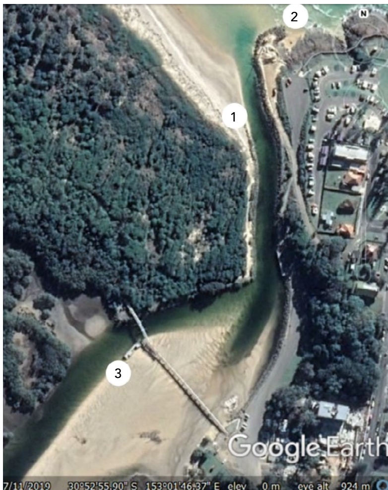
South West Rocks Creek in 2019 with (1) northern breakwater; (2) southern breakwater and commercial drag-line dredging operation work area; (3) fishing pontoon with access for people with disability Credit: Google Earth
