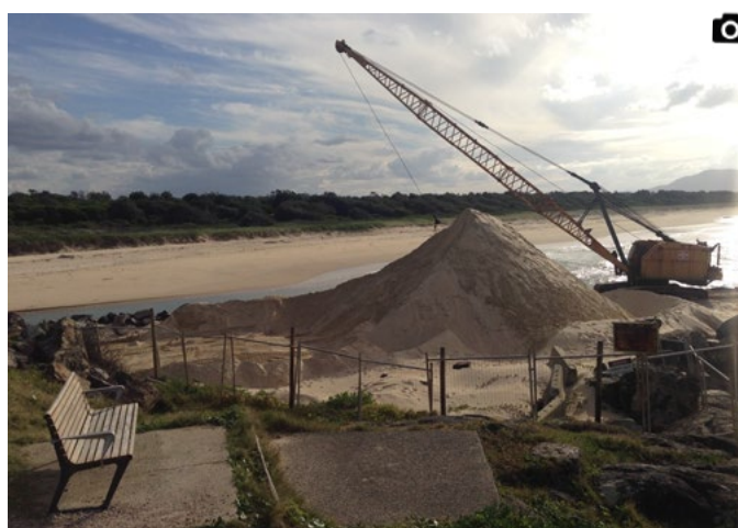
Commercial drag-line dredging operation in South West Rocks Creek
