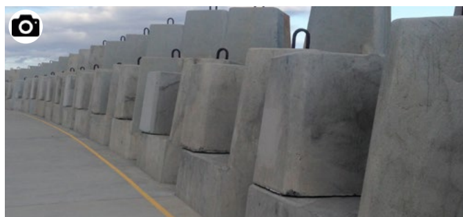
Concrete Hanbar units with attached lifting hooks on the eastern breakwater limit opportunities to enjoy the view to the south east over Korffs Islet
