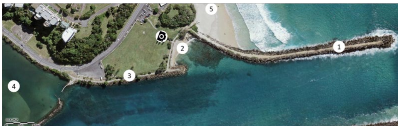
Northern Tweed River Breakwater: (1) the breakwater extension completed in the 1960s; (2) wave-trap beach; (3) original breakwater now part of estuarine training wall; (4) Jack Evans Boat Harbour; (5) Duranbah surf beach
