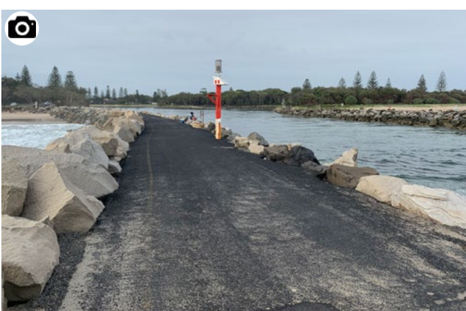
Tarred surface of the breakwater
