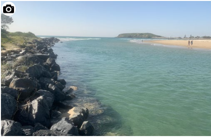
Shifting sands in Coffs Creek sometimes bury the northern training wall and expose it at other times.
