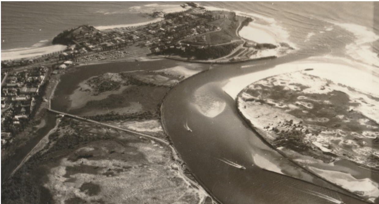
1961 aerial photo of the Jack Evans Boat Harbour formed by training walls at the entrance to the Tweed estuarine Credit: NSW Public Works
