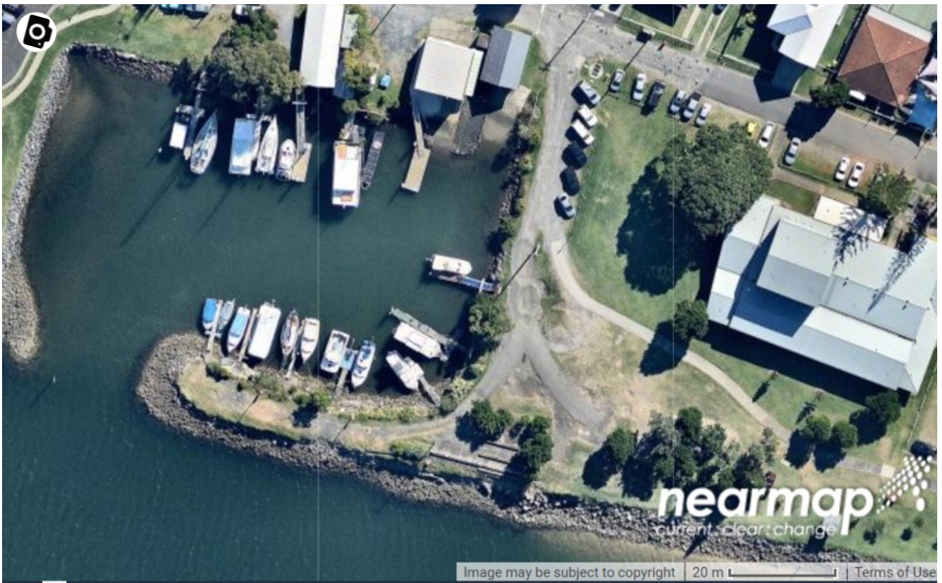
The Martin Street Boat Harbour was formed as part of the Richmond River estuary training walls. Credit: nearmap
