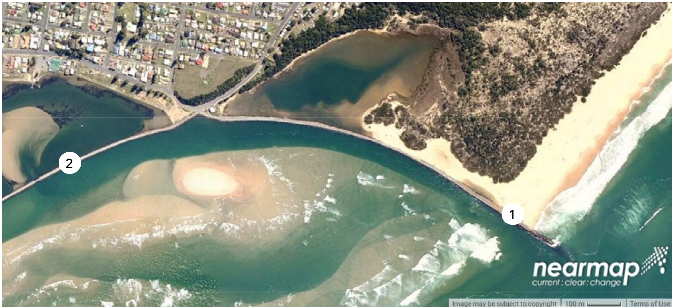
Aerial photo 2011 of the Manning River northern breakwater with the river following the training wall Credit: nearmap
