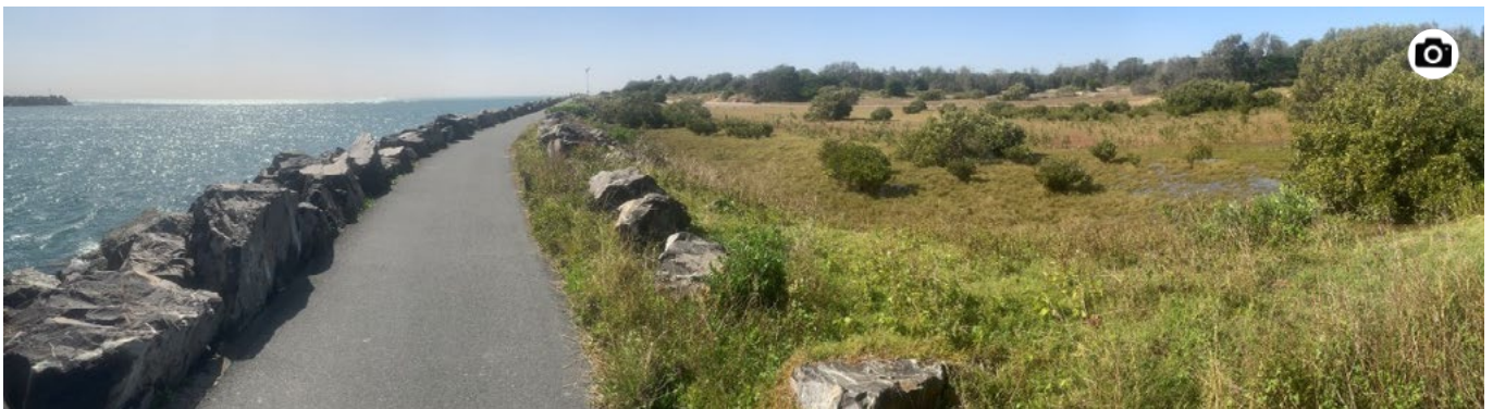
Macleay southern breakwater with saltmarsh and mangrove habitats landward of the structure reliant on flows through the wall
