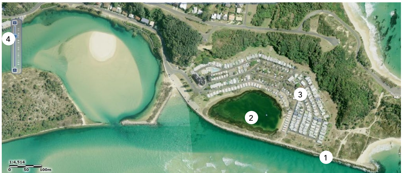
The Nambucca Northern breakwater: (1) northern breakwater; (2) sea lido; (3) caravan park reliant on the training wall; (4) the Glen, Inner Harbour and Freshwater Creek Credit: Six Maps
