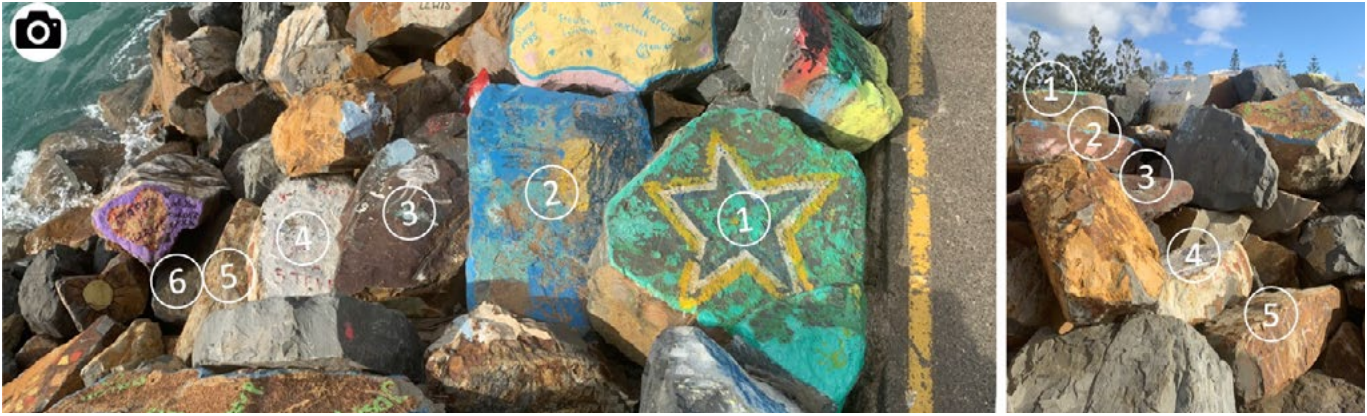
Emergency safety stairs created through careful rock placement during maintenance of the Hastings southern breakwater
