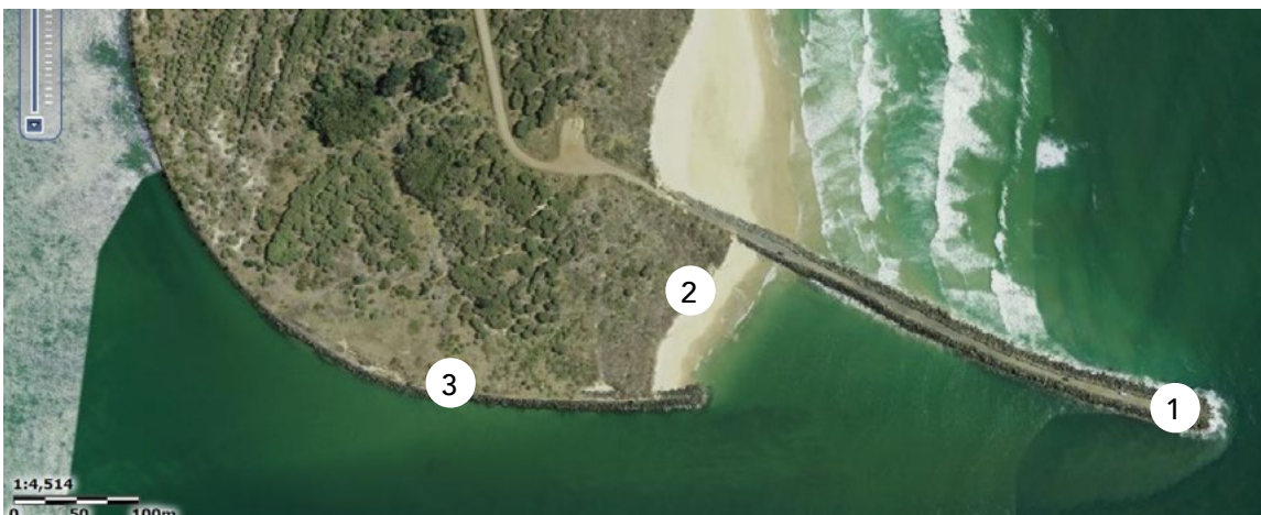
Hastings River Breakwater: (1) northern breakwater built in 1979; (2) wave-trap beach; (3) original breakwater built in the 1930s Credit: Six Maps
