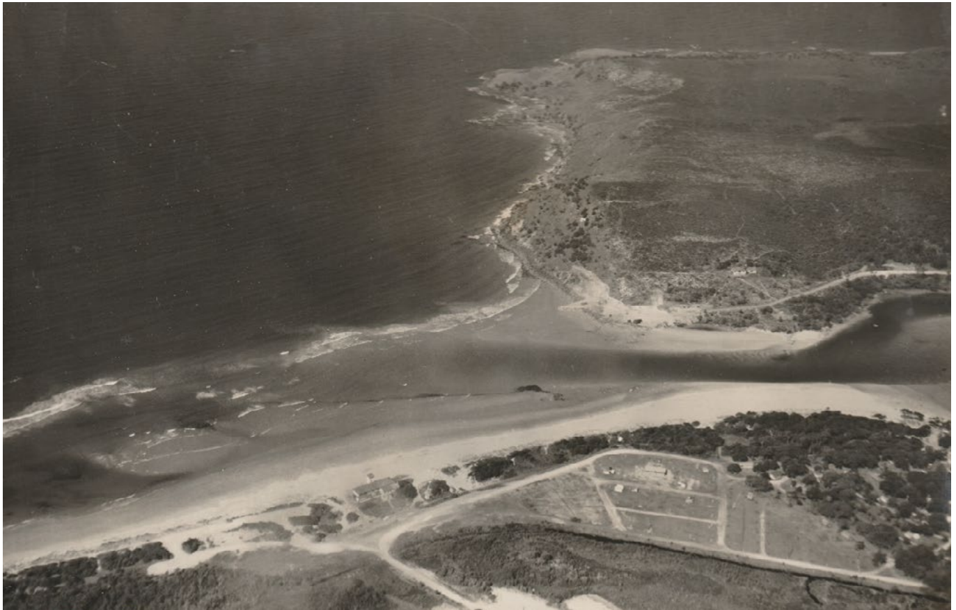
Evans River estuary entrance in September 1960 before the trained entrance was installed Credit: NSW Public Works
