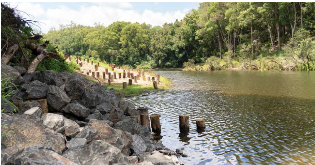
Photo 1. Completed restoration works on the Tweed River, stabilising the river channel supporting natural recovery, following devastating floods in 2022. Credit: NSW Soil Conservation Service
