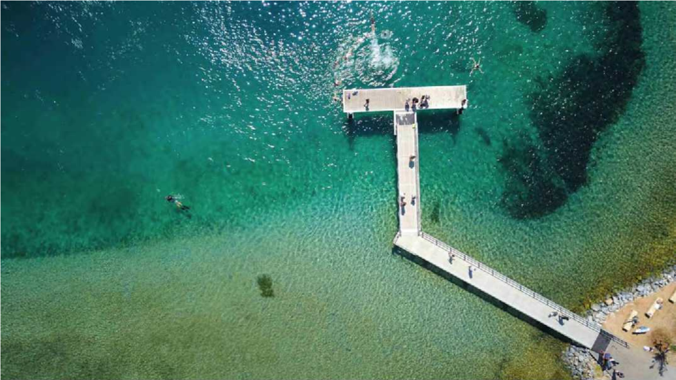
Photo 3. Aerial image of the jetty and pontoon installed as part of the Wagonga Inlet Living Shoreline Project that was officially launched in February 2025 at Narooma, NSW. Credit: Tideline Productions.
