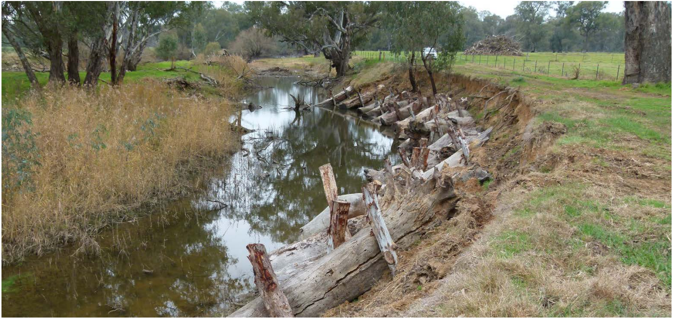
Photo 2. River bank erosion control and stabilisation. Photo: DPI
