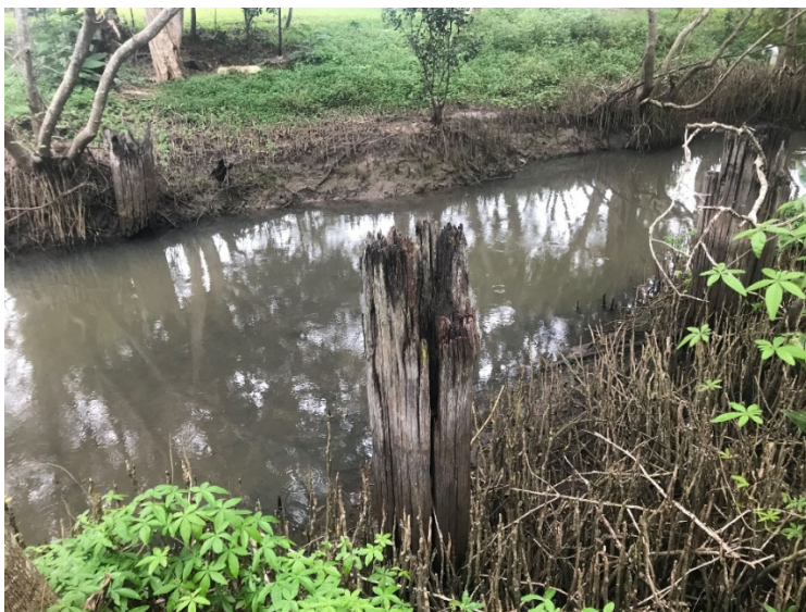
Jarrett Creek bridge piles
