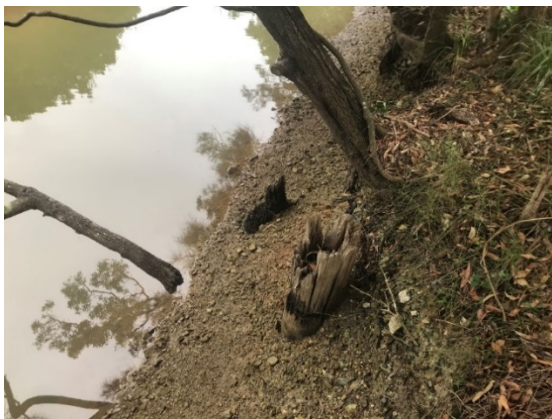
Poundyard Creek bridge piles
