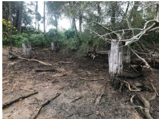
Woolgoolga Creek bridge piles
